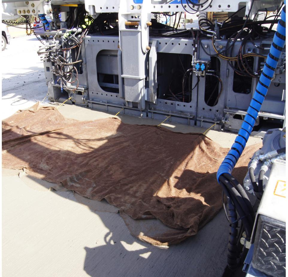
G&Z's Paving Kit includes a deep section frame that is rigid enough to easily span the S400 design width and achieve excellent smoothness results on projects with strict smoothness requirements. It can be provided with a crown section. The Paving Kit design requires fewer bolts per section allowing for rapid paving width changes. The Paving Kit can be mounted in multiple locations under the S400 Tractor and can be quickly and easily mounted or removed from the tractor.
